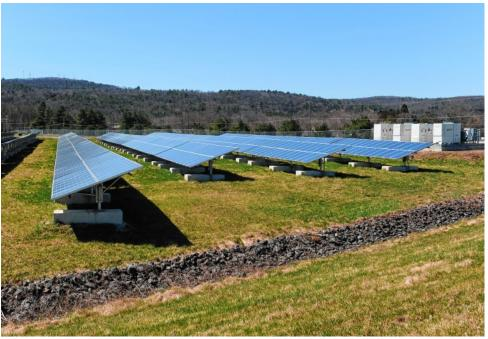
A 2MW solar array on the City's capped landfill has been in operation since 2012 and generates equivalent to half of the municipality's energy use.
